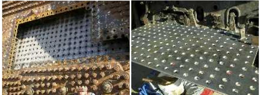
*WELDING TASK #1: Fill the hole in the side sheet (Left) with the tediously prepared patch (Right). High quality welding is critical.*
