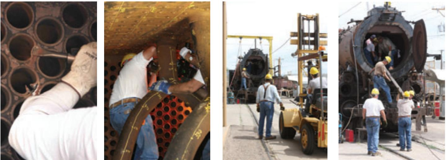
*Tube removal steps: 1: Working in smokebox to collapse swaged tube at front tube sheet. 2: Working in cramped firebox space and using internal cutting tool to cut firebox end of tube. 3: Using forklift and cable to pull tube. 4: First tube removed from smokebox.*
