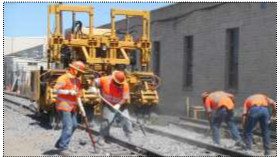
Men & Machine: Gandy Dancers and "Henry"* make short work of leveling ballast on the new track. *Everything at the site gets a name after a while. Henry might be named for one of our favorite viola players.
