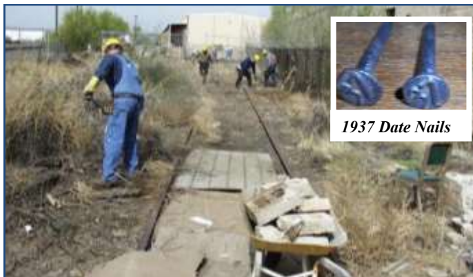
Early 2002: There's Gotta Be A Spur Under Here. A lot of work, but not on a locomotive. Inset shows date nails removed from ties.
