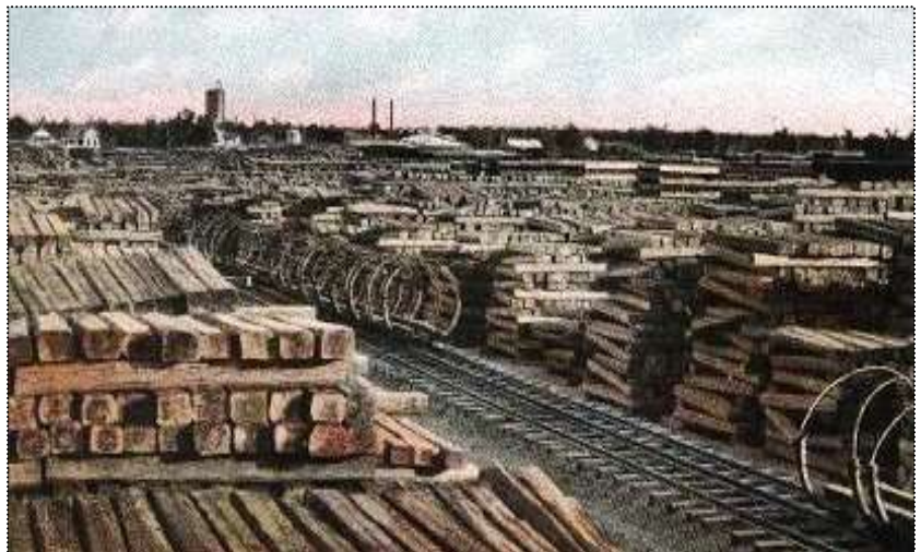
Somerville Tie Plant Circa 1900. It is still operating today.
