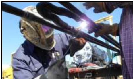
This picture, shot from below the superheater assembly table shows welding underway on a superheater pair with the front of 2926 visible in the background. The superheater welding must be high quality. For the welder, it involves a lot of bending and twisting.
